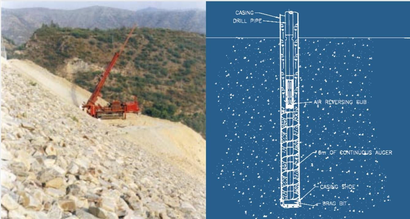
Foremost DR-24 working at dam site. Because of concern over blowout potential, an air-reversing sub was positioned 6m (18ft) above the drill bit to divert air flow back up the annulus to clear cuttings from the auger string. The tooling configuration created a low-pressure vacuum at the bit, eliminating the possibility of a blowout.
