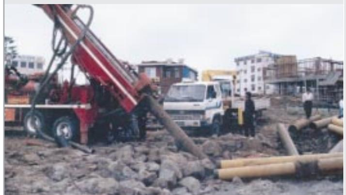
Foremost DR-24 drilling and casing at 45-degree angle
